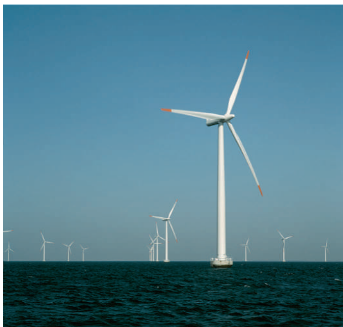
16 Application example, offshore wind turbine
